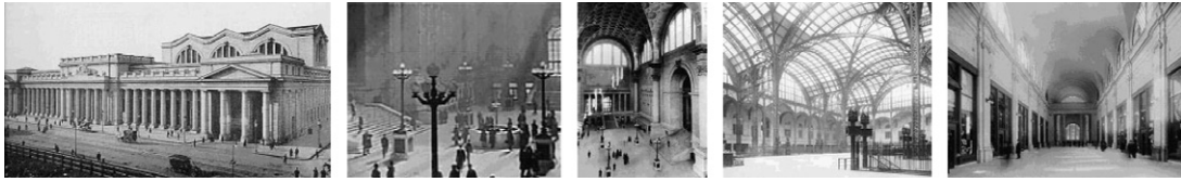
Fig. 2. Historical photos of the original Pennsylvania Station in New York City.
